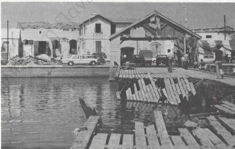
The results of Turkish "police" action. The jetty and customs warehouses at Paphos port, damaged by Turkish air attacks.
