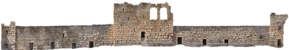
Figure 4. Rectified images of the western internal façade of the Azraq castle.
