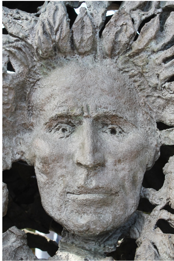
Before work began. Notice the discoloration and build up due to the elements.
