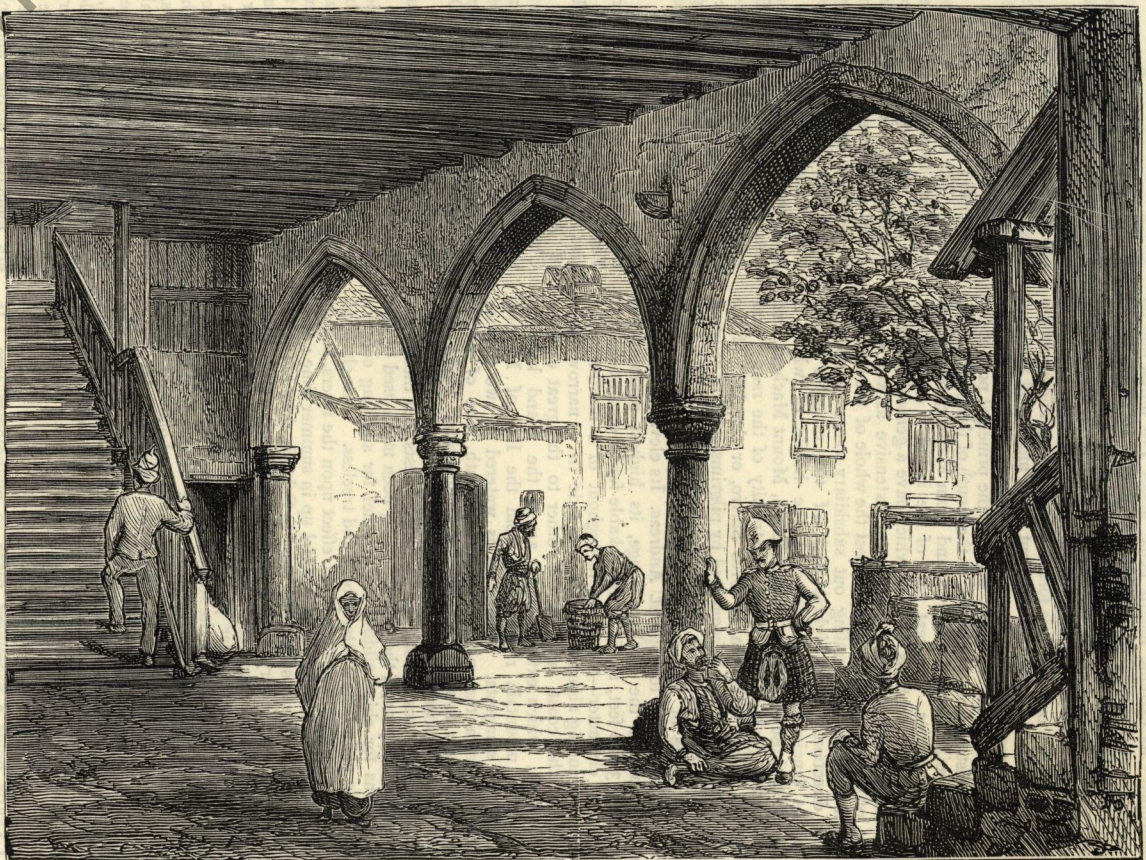
COURTYARD OF THE BRITISH CONSULATE AT LARNACA
