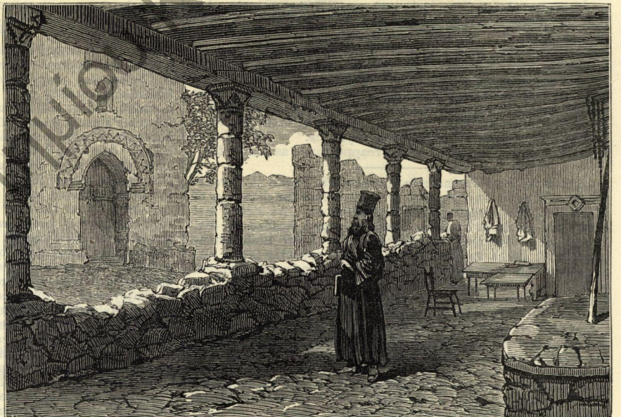
CLOISTERS OF MONASTERY, KANTARA.
