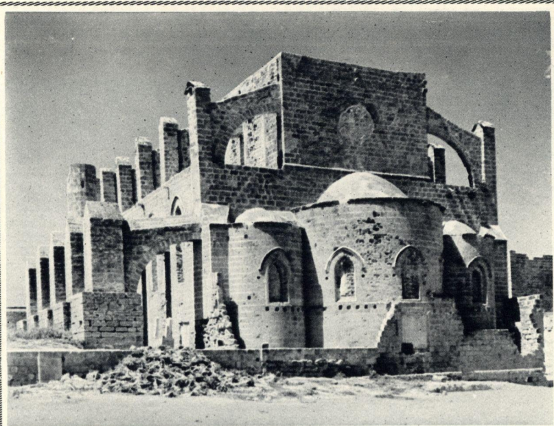
THE CHURCH OF ST. PETER AND ST. PAUL, BUILT ABOUT 1360 BY A MERCHANT FROM HIS PROFITS : THE EAST END.
