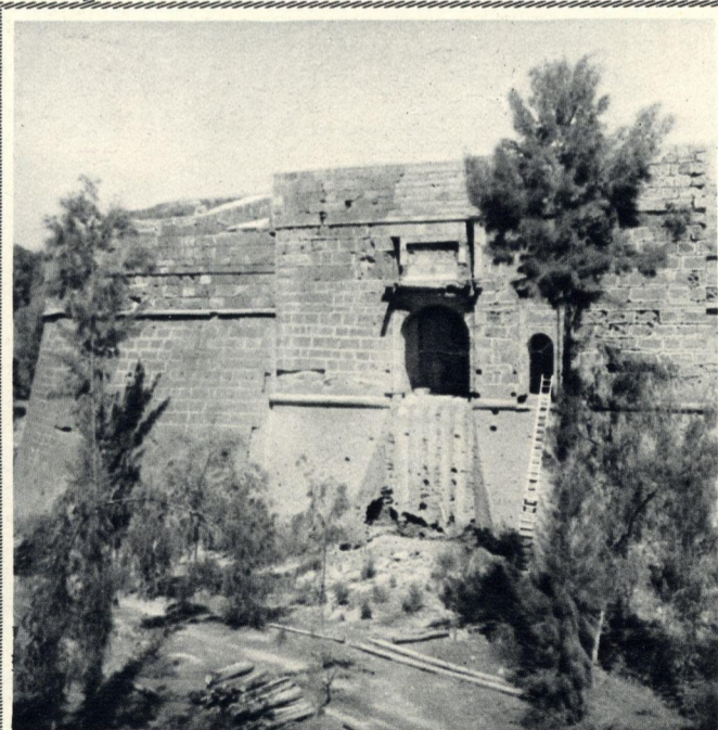
THE GREAT RAVELIN AFTER TREATMENT—FOR COMPARISON WITH THE PHOTOGRAPH ON THE LEFT : THE FORMER GATES REOPENED, AND A PATCH PUT ON ABOVE THE MAIN ARCH.
