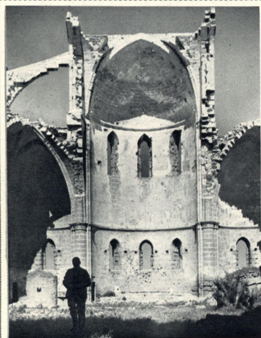
THE CHURCH OF ST. GEORGE THE GREEK : THE EAST END, WHICH HAS BEEN SECURED AGAINST FURTHER DISINTEGRATION.
