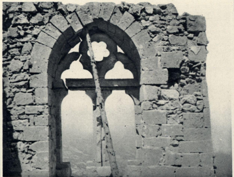
A WINDOW IN THE MOUNTAIN CASTLE OF ST. HILARION: VOUSOIRS PROPPED IN PLACE.
