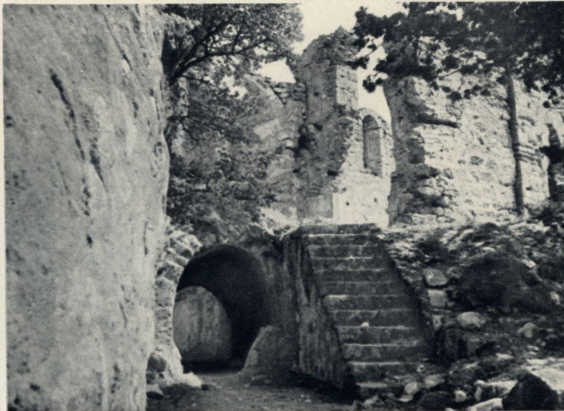
THE NEED FOR WORK OF PRESERVATION AT ST. HILARION: A COVERED STONE PASSAGE, NOW OPEN THROUGH THE FALL OF THE BARREL VAULT.
