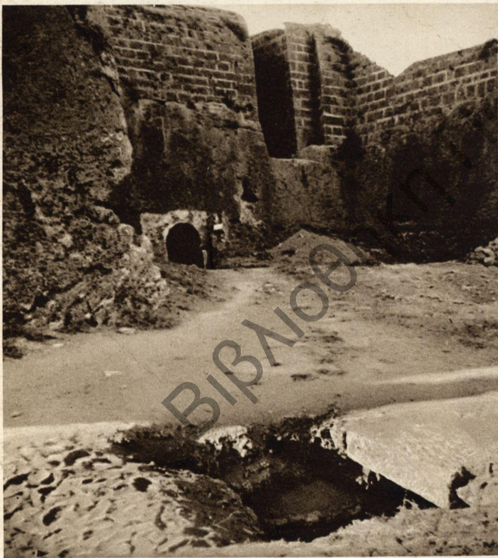
THE SOUTH FLANK OF THE MARTINENGO BASTION, FAMAGUSTA; SHOWING THE SALLY PORT, AND (IN FOREGROUND) AN OPENING IN THE CEILING OF AN UNDERGROUND PASSAGE.
