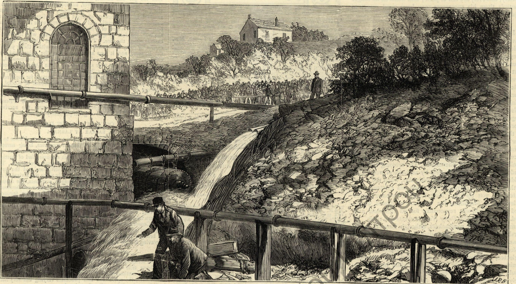
THE ABERCARNE COLLIERY DISASTER—TURNING THE CANAL WATER INTO THE PIT
