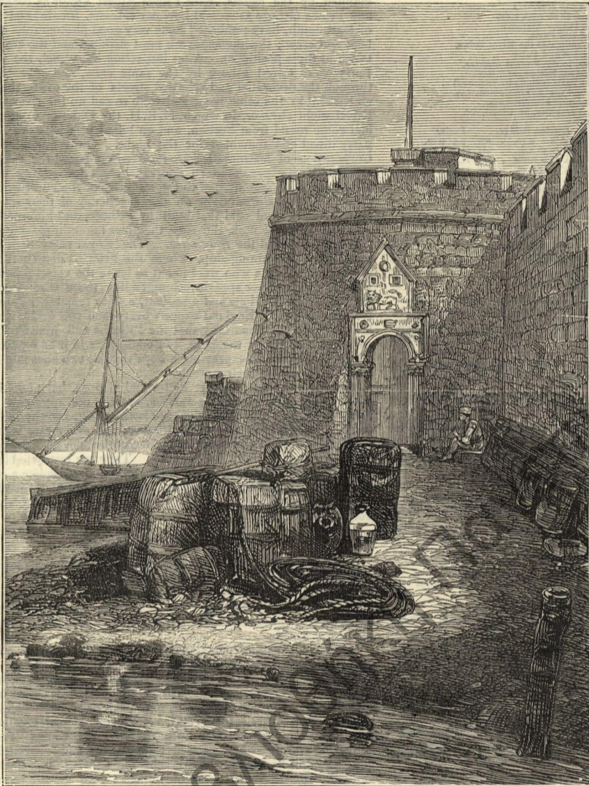
WATER GATE AT FAMAGOSTA
