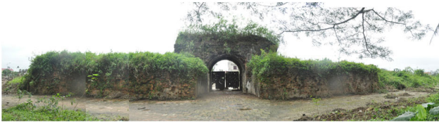
Figure 4: East gate front of Quang Tri citadel
