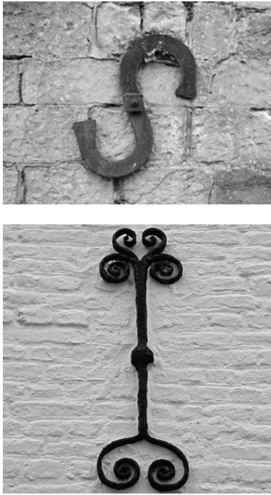
Figure 6: Traditional Gothic tie rod anchors
