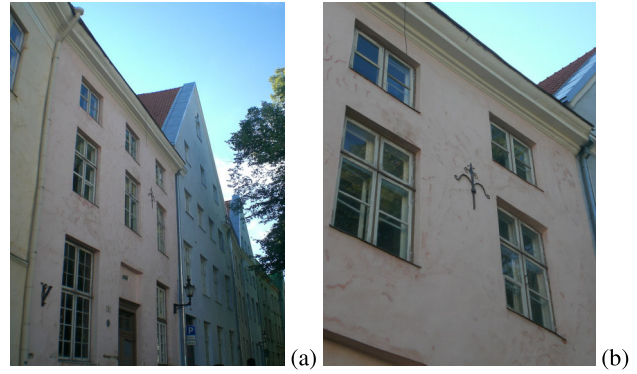
Figure 8: Tallinn: retrofitted building in old town (a), tie rod anchor (b)
