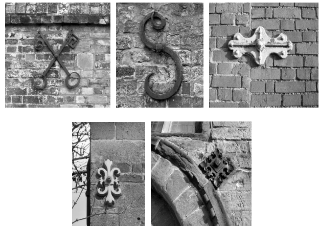
Figure 16: Decorated wrought iron tie rod anchor
