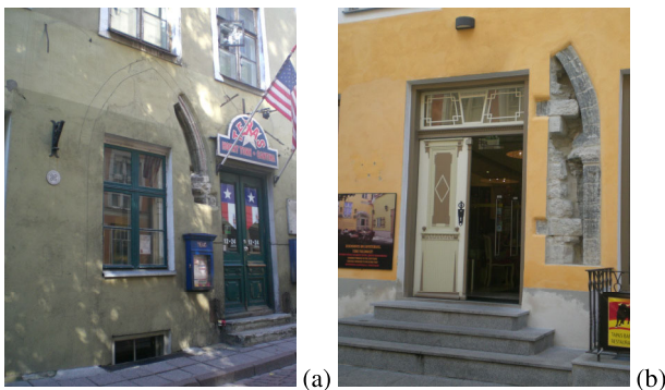
Figure 7: Tallinn: retrofitted building in old town (a), traces of original structure: façade detail (b)
