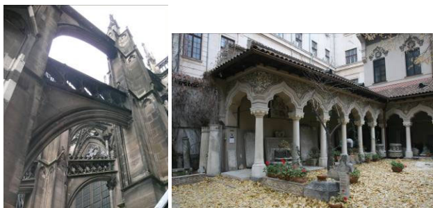
Figure 2. Example of different decay phenomena on outdoor stone materials in two of the selected sites: extensive biocolonization in Cologne Cathedral (Germany) (left) and surface dissolution and erosion on Stavropoleos Monastery in Bucharest (right).
