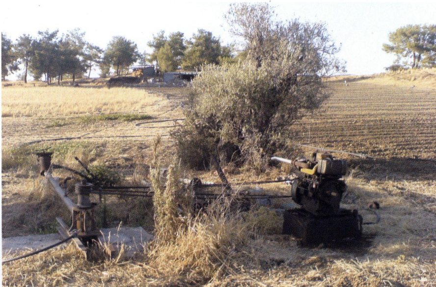
b: One of the many still active diesel pumps for irrigation. Sia-Mathiatis area.
